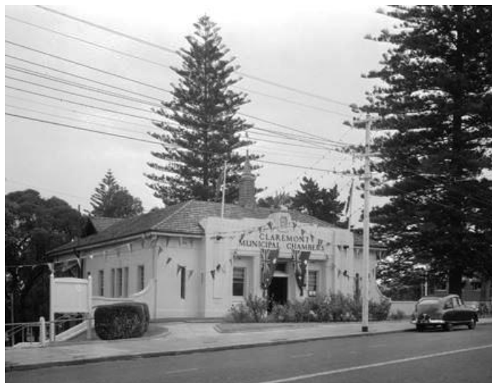
Claremont Council Chambers of 1935, pictured in 1954. The building was significantly damaged by fire in November 2010, but is planned to be rebuilt. (SLWA 102605PD)
